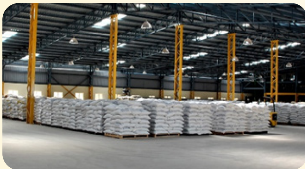
Figure 1: Well ventilated and proper storage
