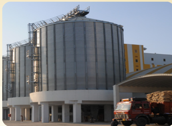
Figure 2: Grain storage silo
